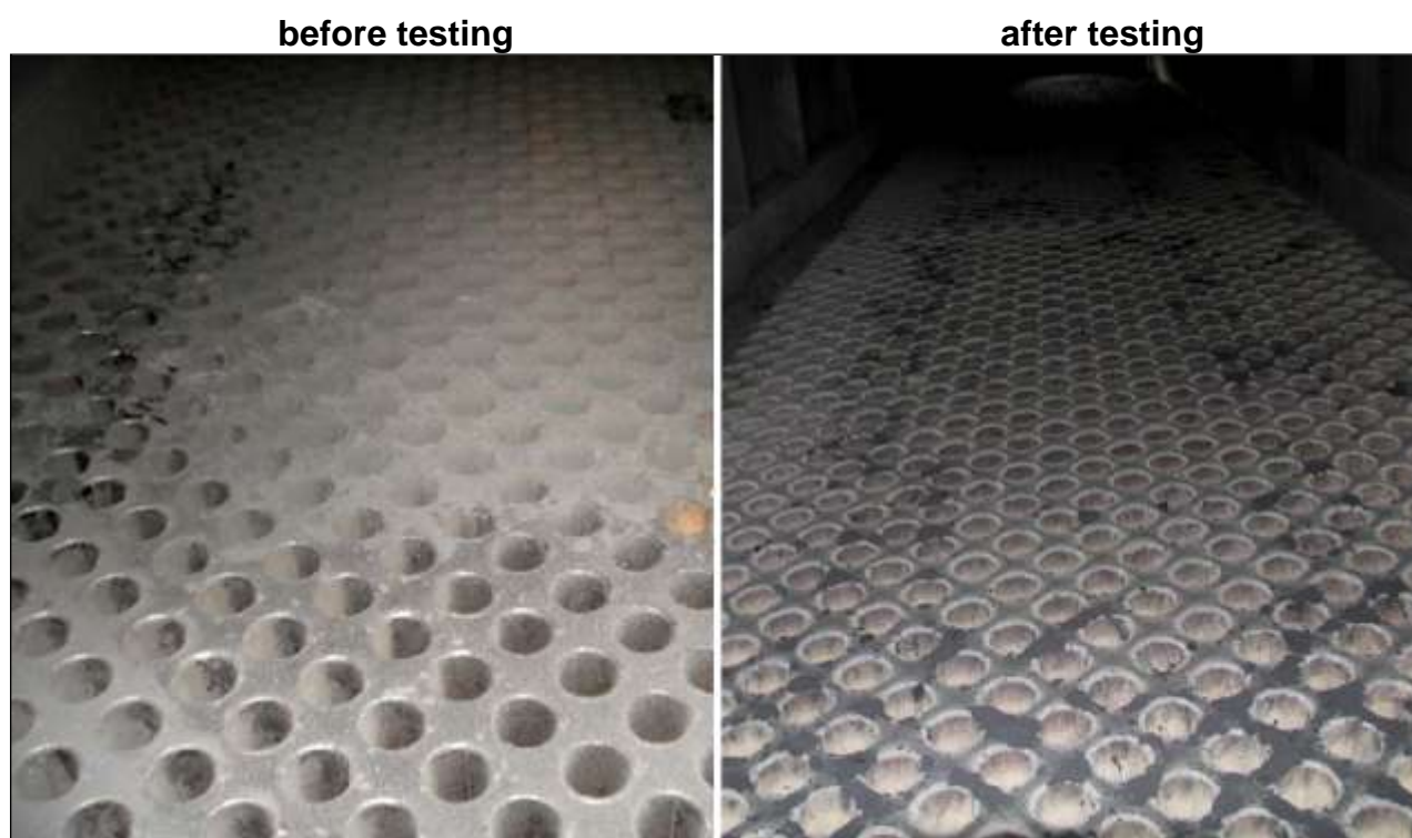
Figure 14 Tubular air heater
