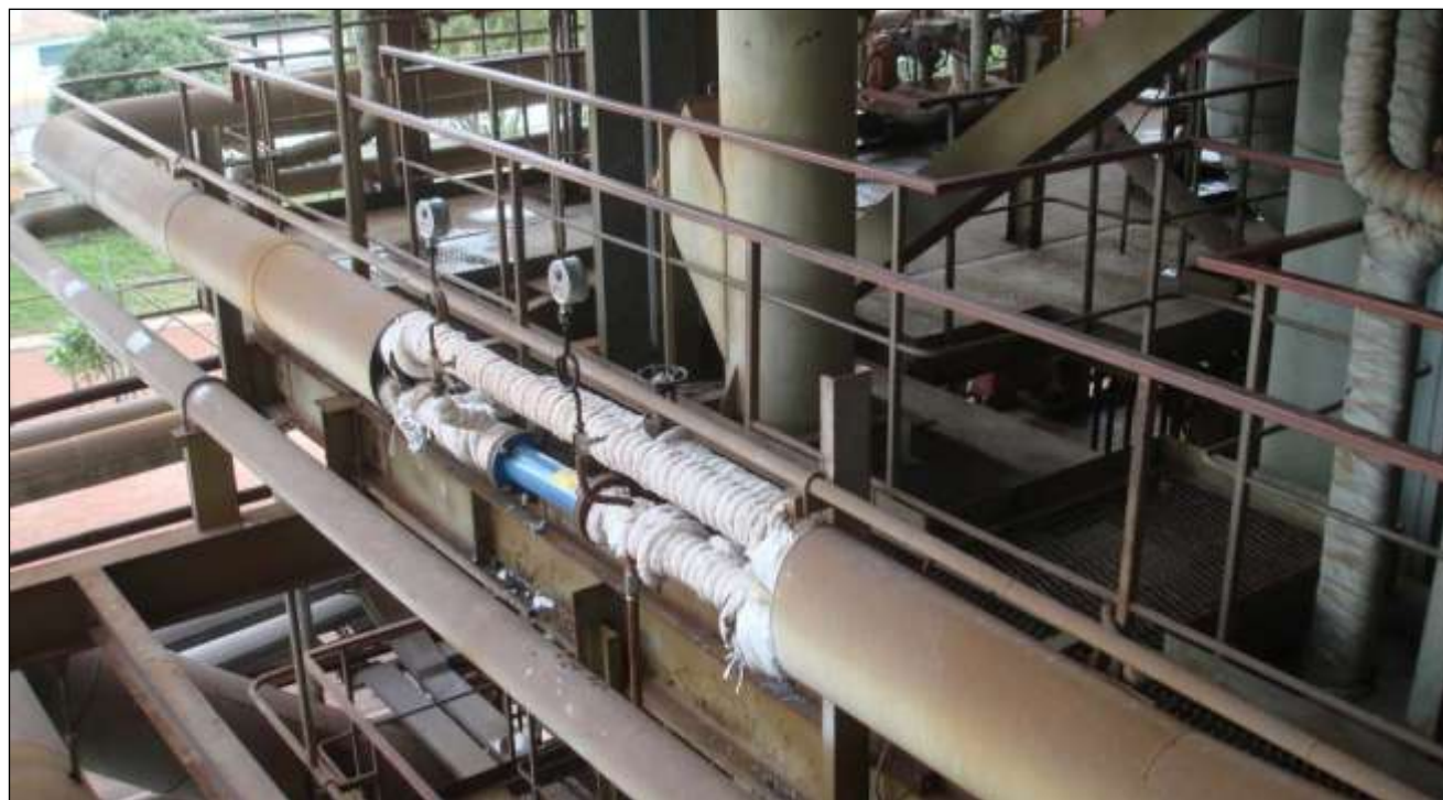
Figure 1 Installation of homogenizer on the boiler 5
