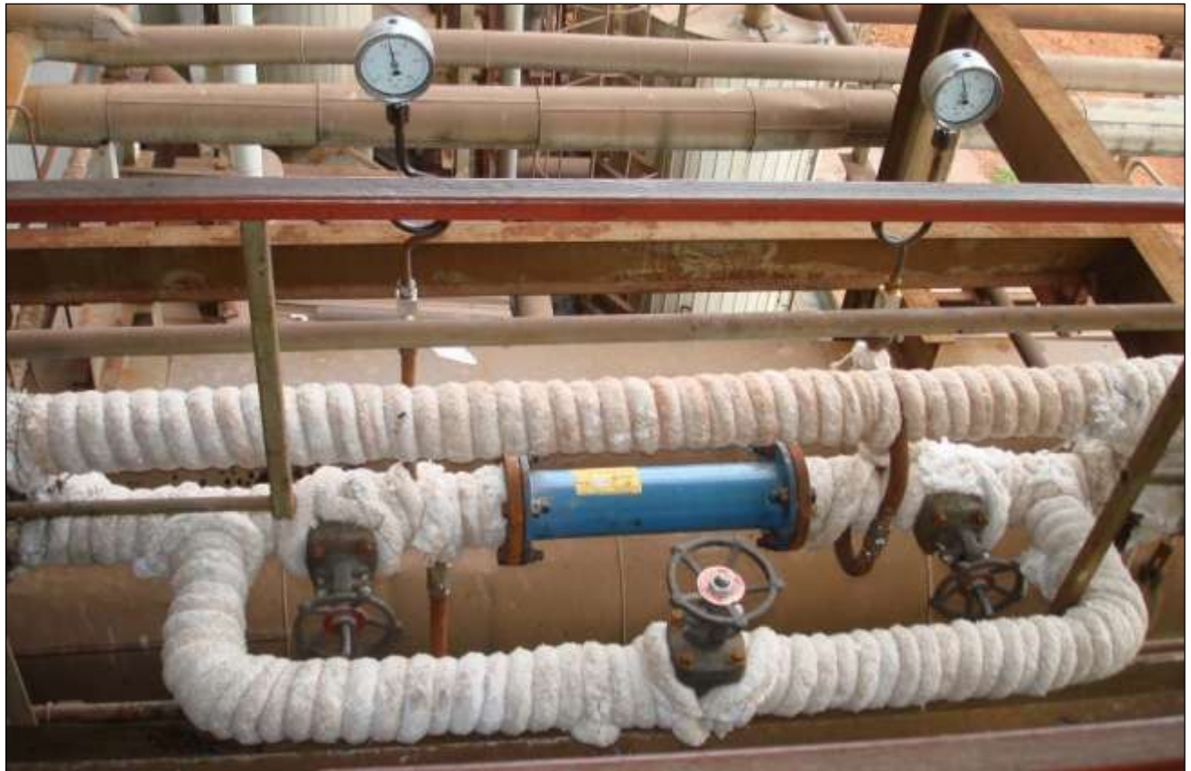
Figure Nr.2 Installation of homogenizer on the boiler 5
