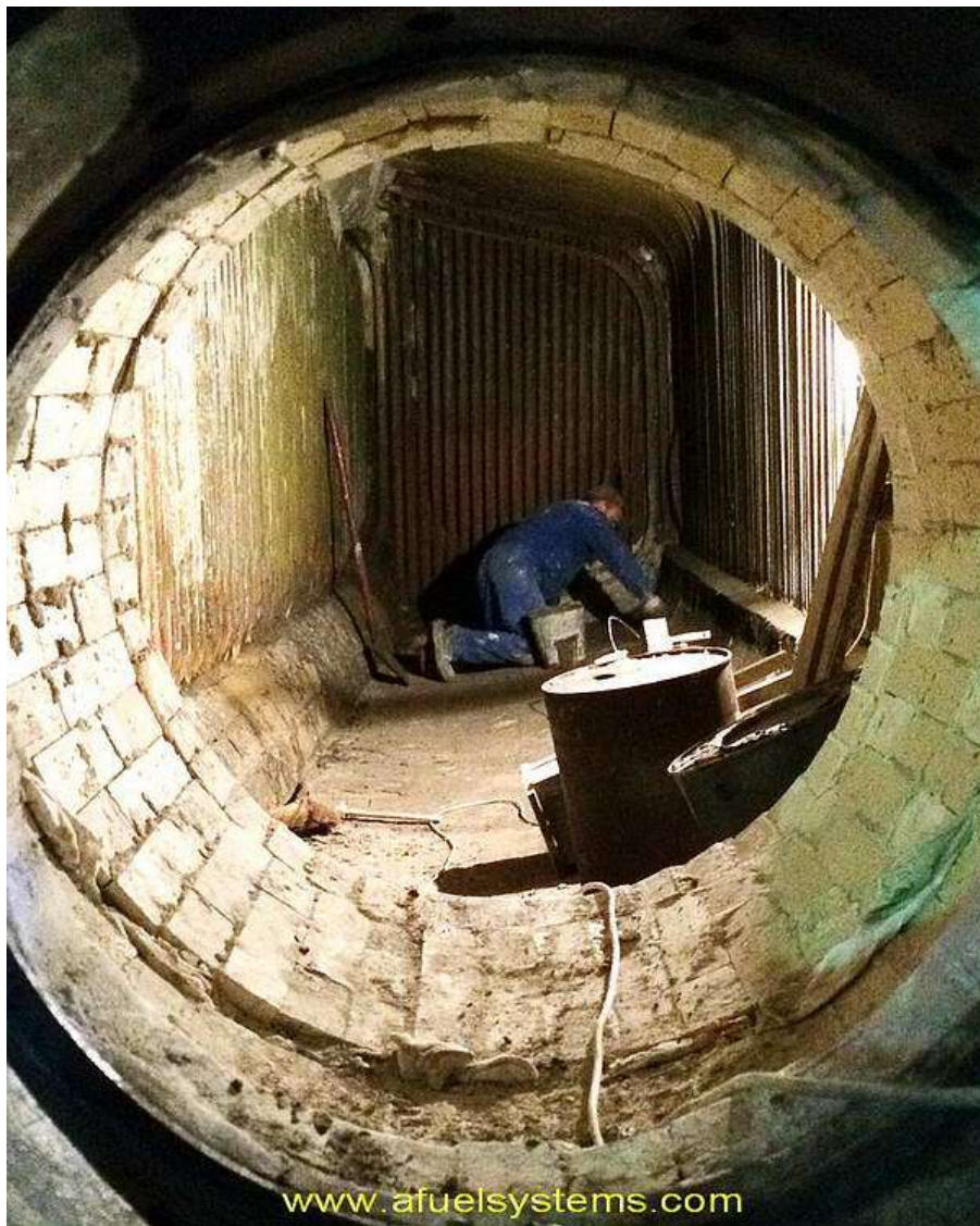
Cleaning boiler "before" – long, hard and mechanical removal of the soot.
