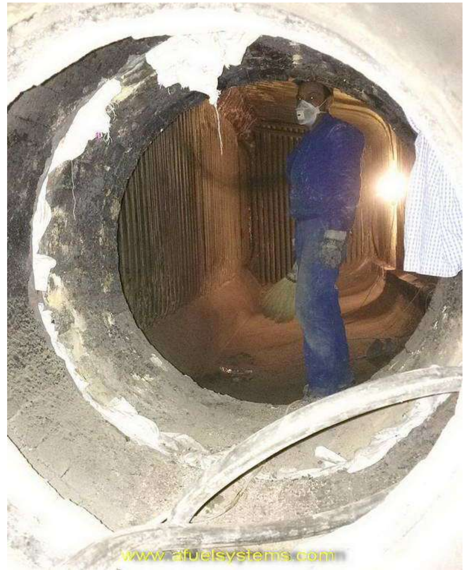
Boiler cleaning "after" - tapping and removing bt broom.
